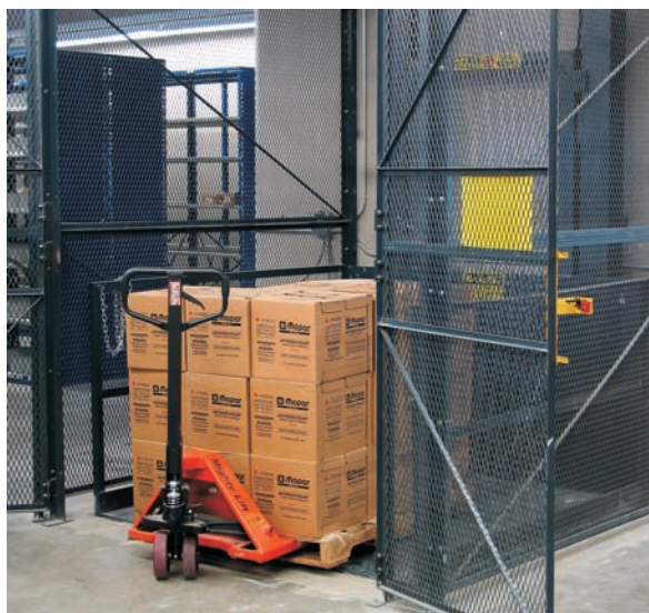
Hydraulic Lifts and Pallet Jacks move items easily between levels.
